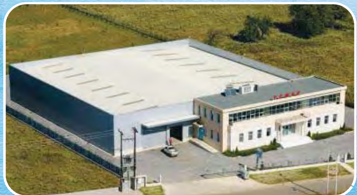
Premises 2.600m 2 THESSALONIKI - NORTH GREECE
